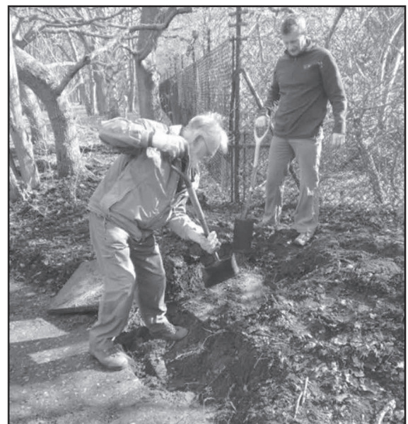
Fixing drainage Photo by S Corley
